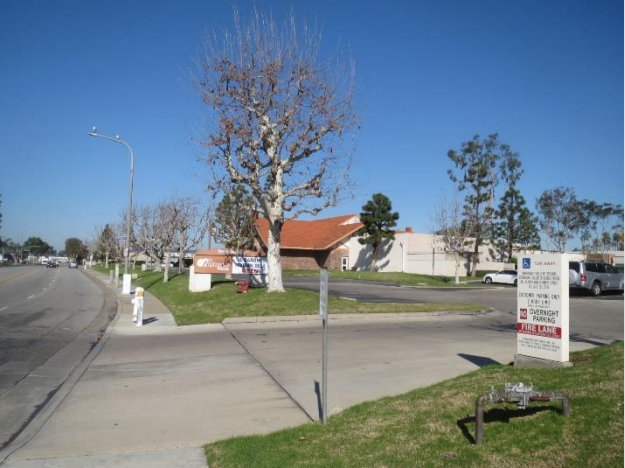
2. View of Property, facing north
