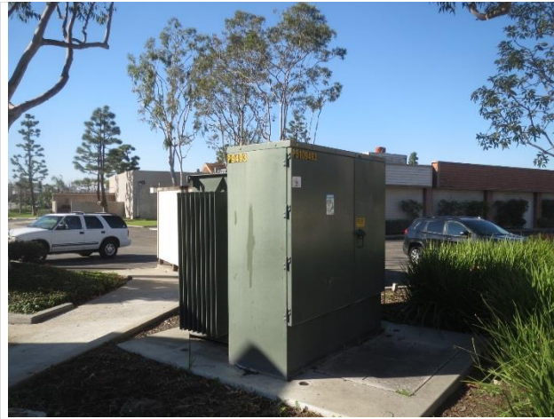
20. Pad-mounted transformer
