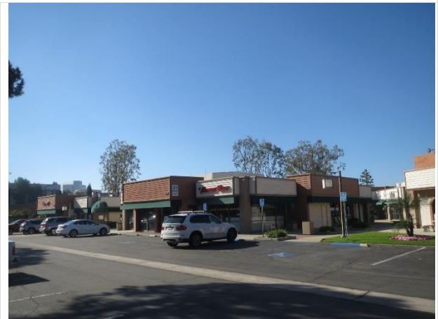
6. View of south side of Property, facing southeast
