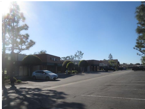
11. Typical tenant entrance
