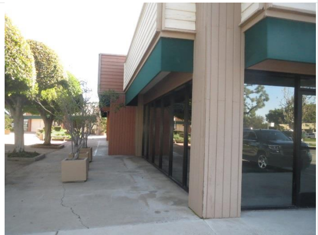
12. Typical common area
