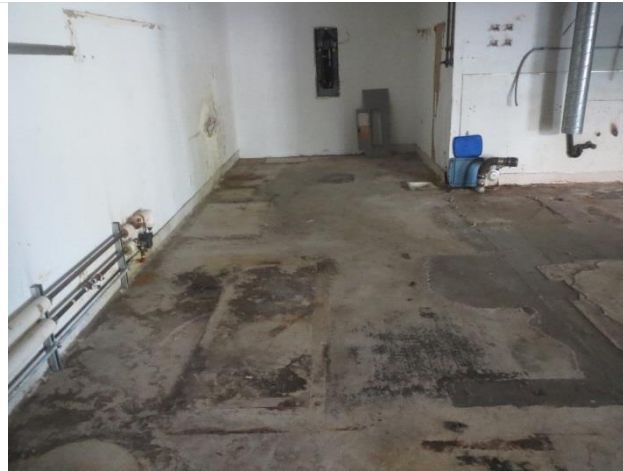
14. Former dry cleaner tenant space – 4250 Scott Drive
