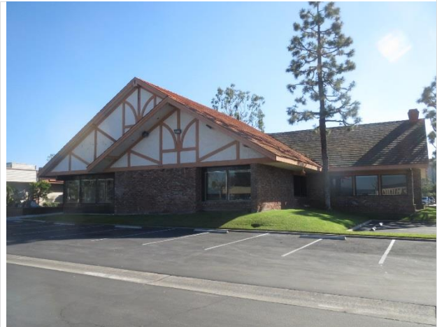
4. View of south side of Property, facing southeast
