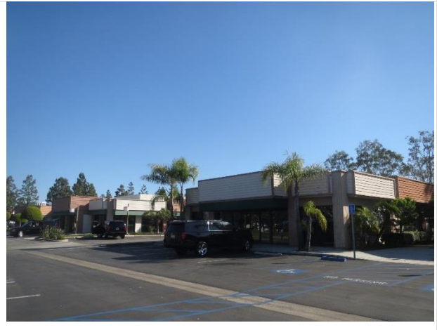
10. Outdoor storage area
