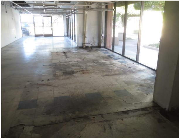
13. Former dry cleaner tenant space – 4250 Scott Drive
